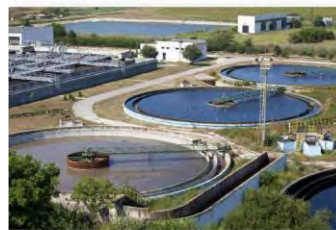
Water Purification Plant
